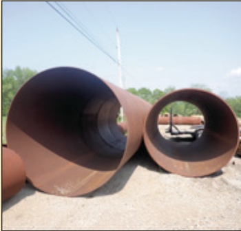
INVENTORY OF FOUNDATION PIPE
